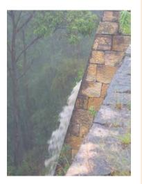
Top: buttress, Devines Hill, viewed from below, was built as a **culvert** to keep water away from road. Above: the same buttress in a rain storm seen from the road
