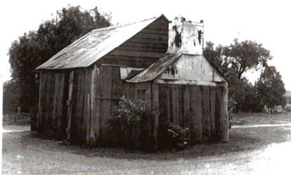
Typical Black Creek slab hut with stinging bark roof replaced with corrugated iron
