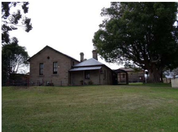
Wollombi Court house built in 1866 of locally quarried stone, the 1890s exercise yard is visible at the side. Photo E.A. Roberts
