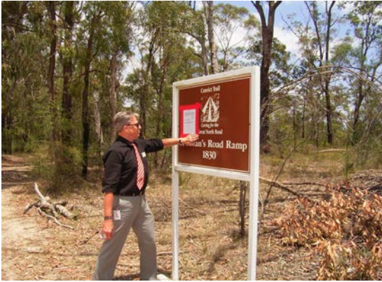
2006 Bill Nethery of NSW Heritage Office installing cease demolition sign in at St Albans Road Ramp
