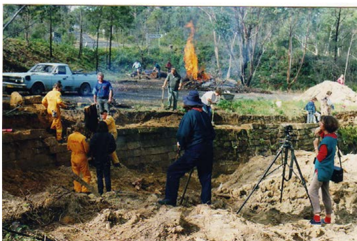
Community with advice rebuilding the wall at Bucketty Photo Paul Budde
