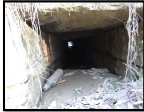
11th Culvert past Native Dog Hill heading towards Cessnock (4) Pipe with stone surround. Below.
