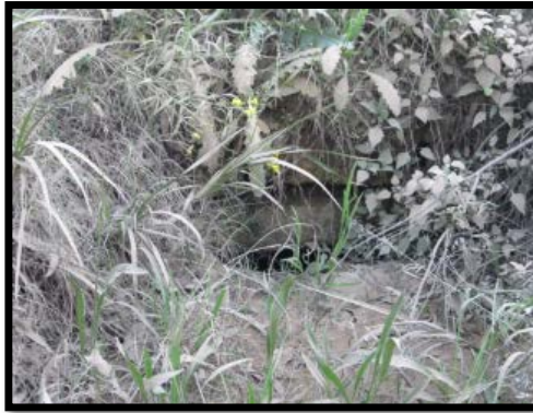
10th Culvert past Native Dog Hill heading towards Cessnock (5)
