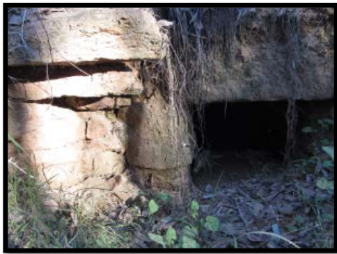
11th Culvert past Native Dog Hill heading towards Cessnock (4) Pipe with stone surround. Below.
